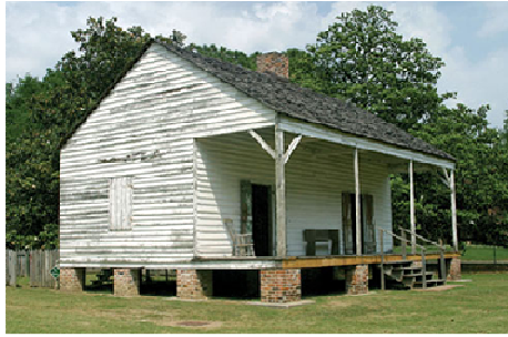
Built up off the earth with clap board siding, a shingled roof, a brick chimney and a window, this later slave cabin would provide much more substantial protection.
